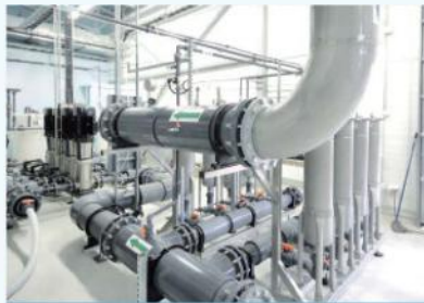
Municipal water supply
